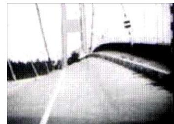
Figure 23-2: The Tacoma bridge disaster is perhaps one of the most well-known failures that resulted directly from resonance phenomena. It is believed that the the wind blowing across the bridge caused the bridge to vibrate like a reed in a clarinet.
